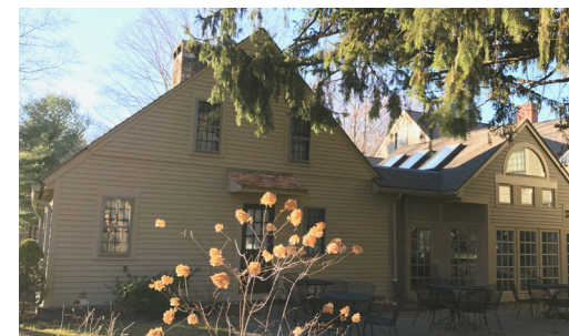
Parmelee House, Sun Room & Patio 2016
