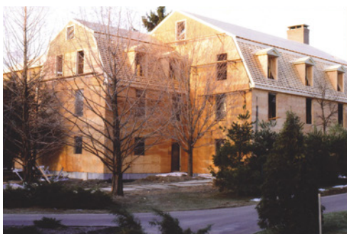
The east wing guest rooms nearing completion
