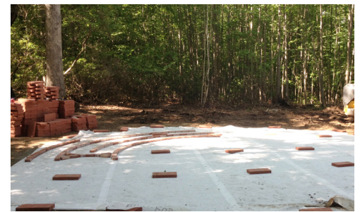
Guest House labyrinth construction, 2013
