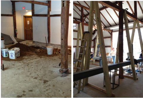
White Barn renovations, 2012
